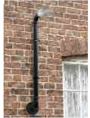
Installed to prevent nuisance pluming across the window
